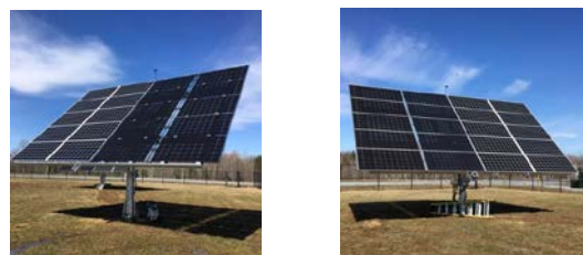
Figure 5: Two axis trackers in Vermont with bifacial and monofacial strings on each.
