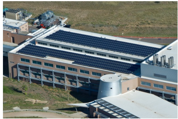
Fig. 4. PV system on the roof of NREL's Science and Technology Facility building which was constructed in 2006.
