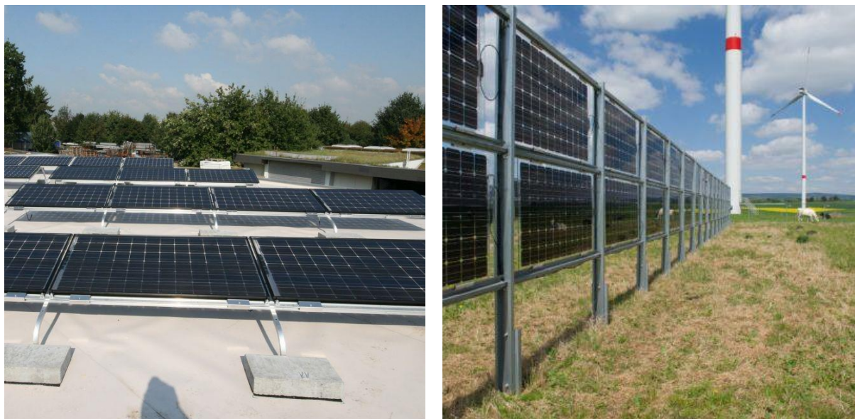
Figure 72: Examples for the two standard mounting conditions selected for bifacial PV module energy rating. Left: fixed installation on a flat roof, tilt angle = 20^\circ , albedo = 60%. Right: vertical east-west facing installation on agricultural ground, albedo = 20%. Photos: Christian Reise, Next2Sun.
