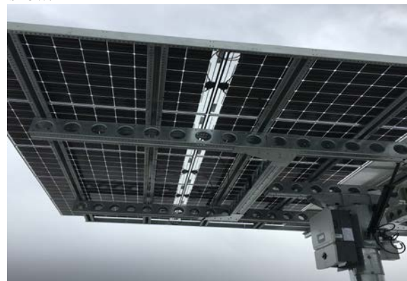
Fig. 13. View of the rear side of the tracker for System 1 showing that support structure blocks the back side of the bifacial modules.
