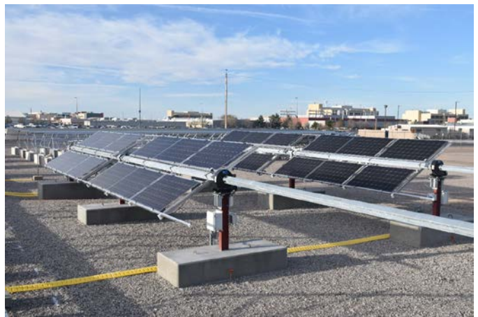
Fig. 4. Single axis tracker for bifacial modules being constructed at Sandia.
