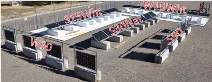
Fig. 2. Bifacial and monofacial modules at five different orientations. Two of the arrays are installed over white rock to enhance back side ground reflections.
