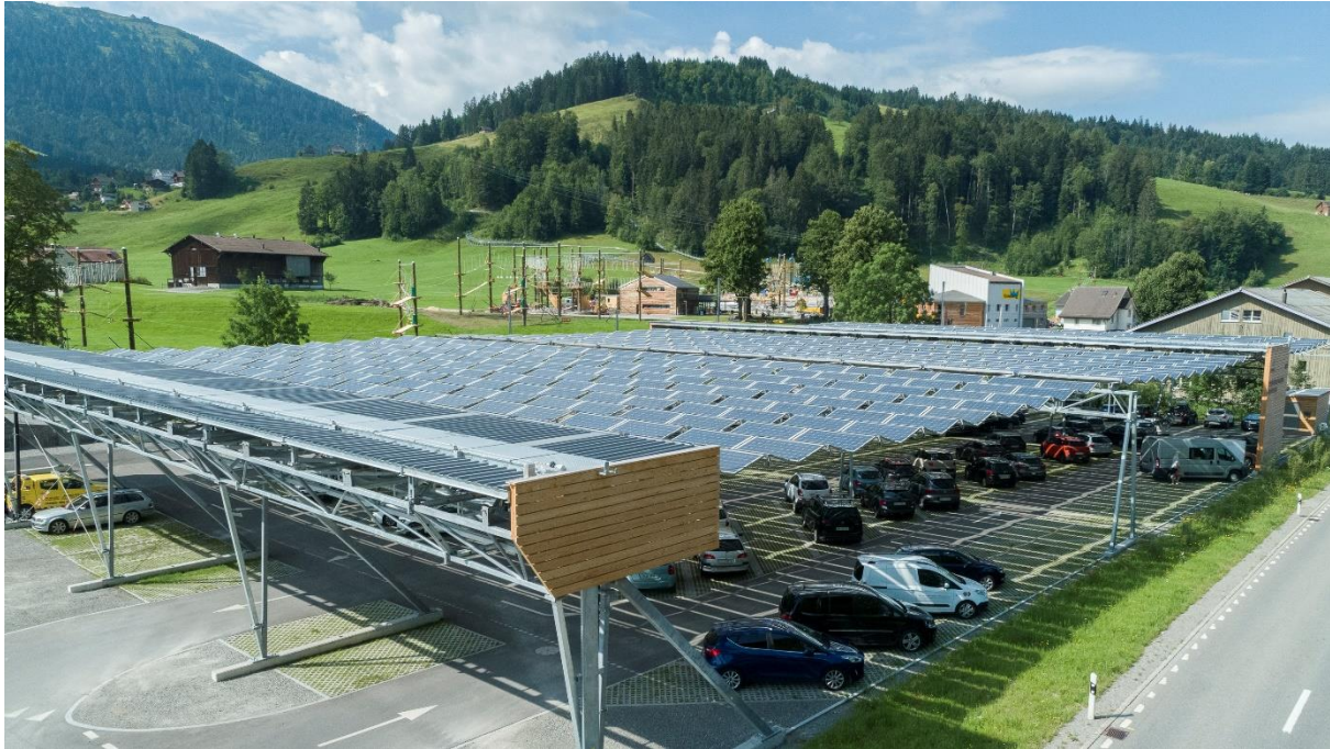
Figure 52: Foldable PV System on top of a carport in Appenzell, Switzerland (Source: dhp technology AG).
