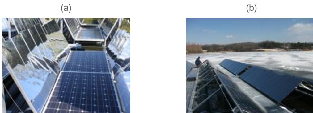
Figure 58: Floating, Tracking, Cooling, Concentrating systems, (a) Colignola-Pisa, Italy [98], (b) Cheongju-si, Korea [98]
