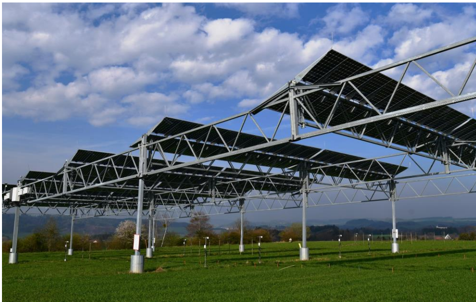
Figure 59: The pilot APV system uses bifacial glass-glass modules arranged in rows of two.
