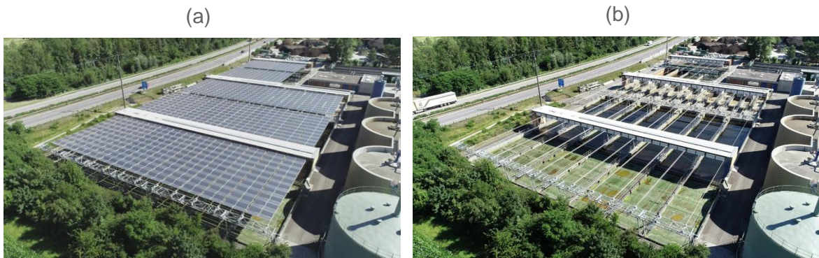
Figure 48: The DHP's 640 kW HORIZON solar foldable PV plant on top of the wastewater retreatment basins in Chur, Switzerland operating since (Source: dhp technology AG).
