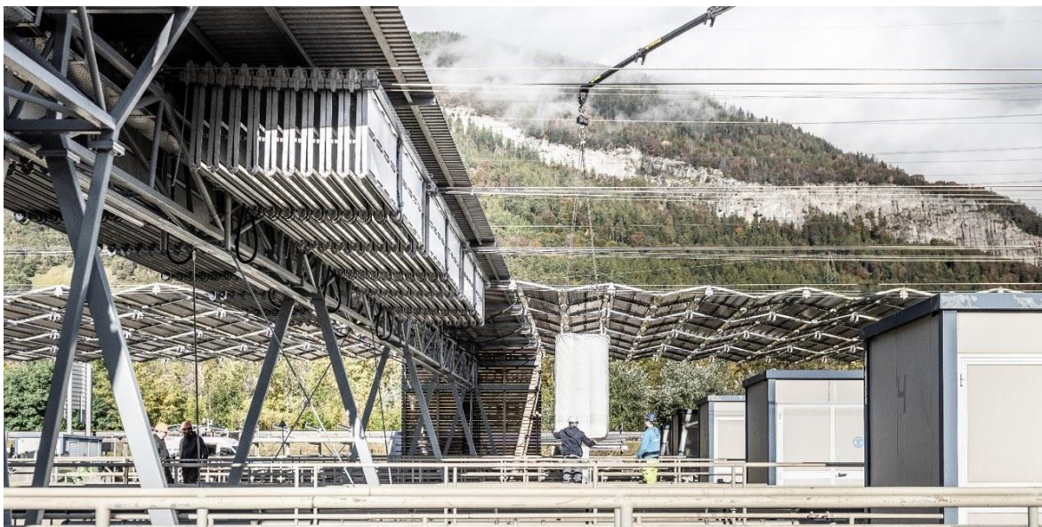
Figure 49: Parts of the PV foldable roof is opened to get access to regular service activities concerning the infrastructure of the wastewater treatment system (Source: dhp technology AG).
