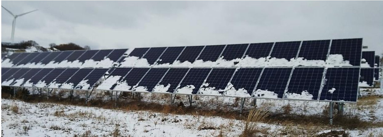
Figure 35: Snow on the PV modules, mountainous landscape, PV power plant size: 20 MWp, Location: Chengde, China, temperate climate.
