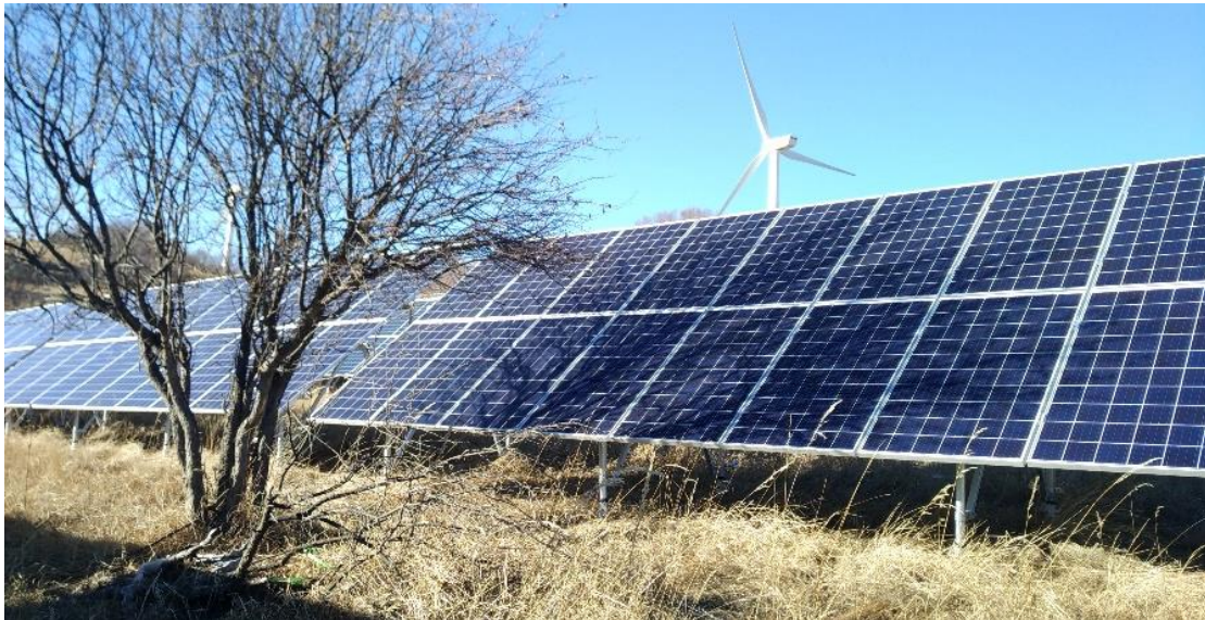
Figure 37: PV system shading by trees.
