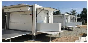
SMA's large scale on-grid project is a 16 MW / 10 MW prequalified PRL (Primärregelleistung – Frequency response) system. The system will be installed within a substation and connected at 33 kV to provide grid stability.
