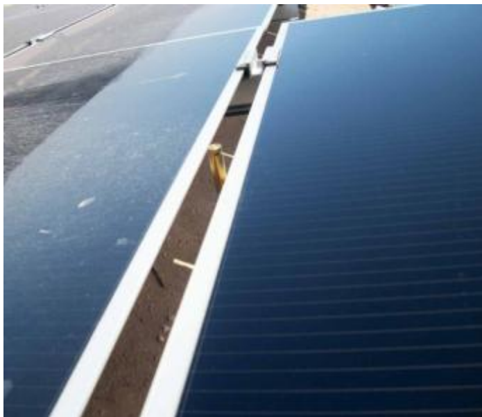
Close-up of water dispensing nozzle, programmed for daily pre-dawn washing
