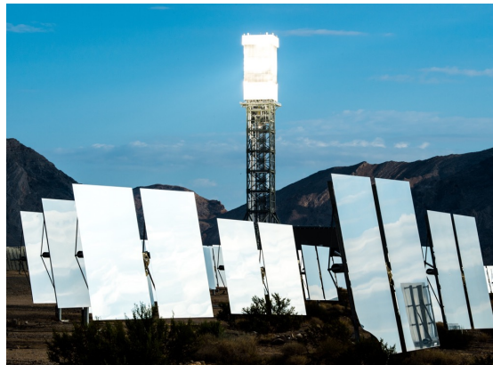
July 26, 2017 - Heliostats at the Ivanpah Solar Project, owned by NRG Energy, Bright Source Energy, Bechtel and Google. (Photo by Dennis Schroeder / NREL)
