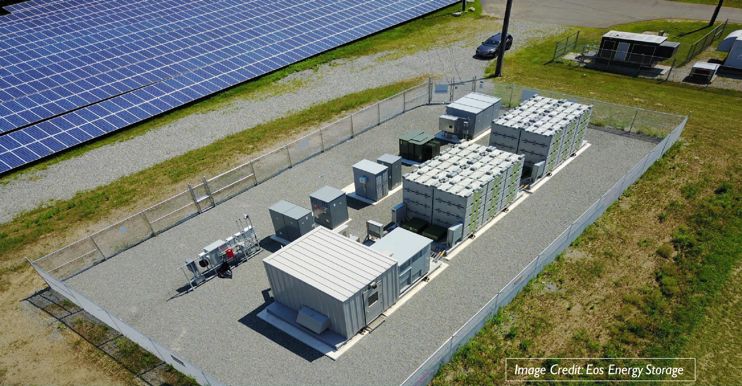
PV + Storage Microgrid for a water treatment facility in Cardwell, NJ
