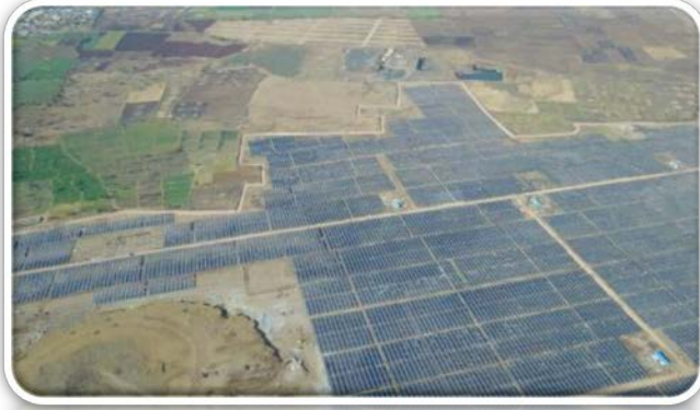
Place: India Time: 2017 Scale: 172MWp
