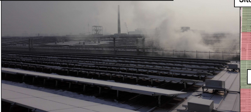
Rooftop Site with Heavy Pollution From Chimney
