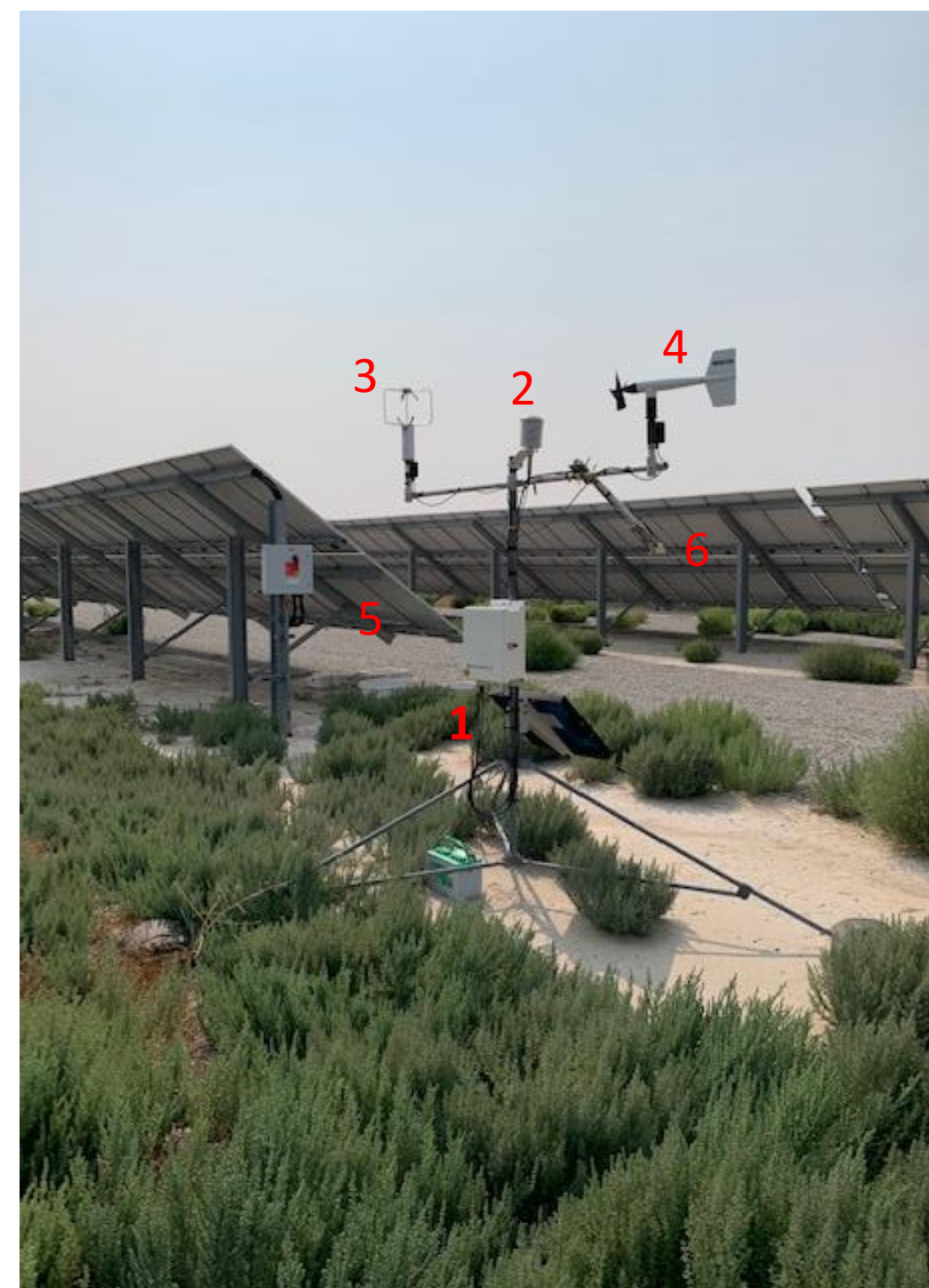
Figure 3: Equipment set up at a station in solar site.
