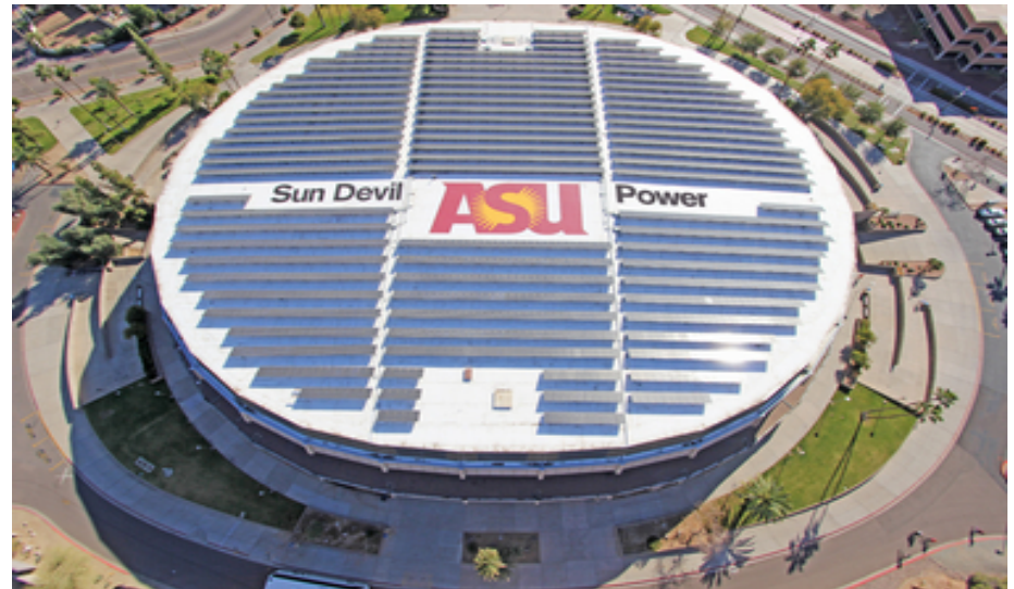
System: 2100 PV modules, 600 – 1500V, 500 kWdc
