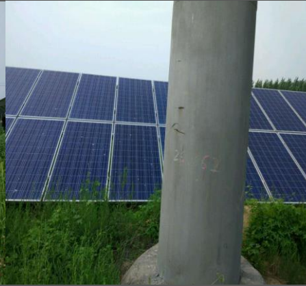
实物遮挡 (Building Shading)
