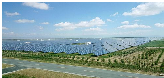
3.2 GW PV station
