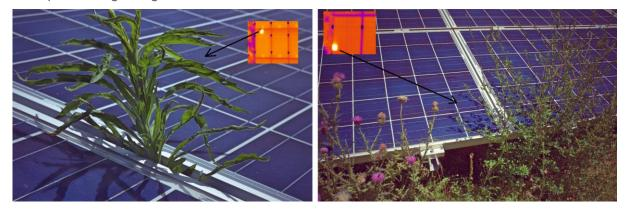
Figure 7: Examples of shading caused by non-managed vegetation at a utility-scale PV plant © CEA-INES.
