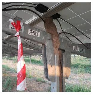
Figure 30: Impact by wildlife on PV components, such as a rat in the main distribution box (left) and termites around the DC cable under the PV module (right).
