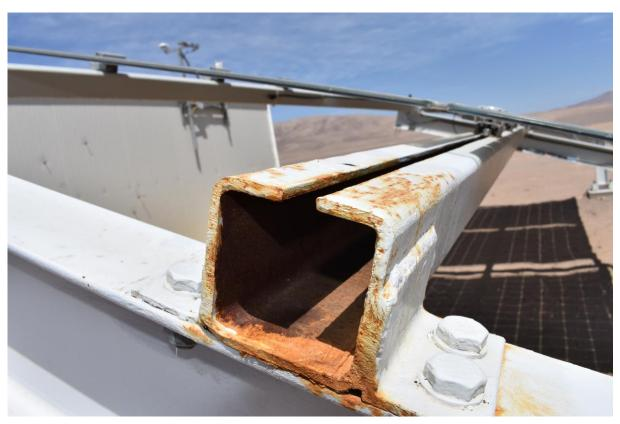
Figure 28: Rusted mounting structure in a PV power plant located in the Atacama Desert. This mounting structure has been in operation for about one year.
