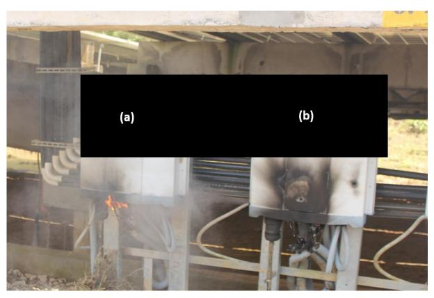
Figure 40: (a) Fire was seen at an inverter several hours after the floodwaters had receded (b) A similar fire probably caused burn marks and failure of several submerged inverters. The manufacturer's name is masked in black.
