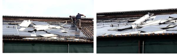
Figure 44: PV System status after a windstorm in Baselga di Piné, Italy. Source: Dino Loriatti.
