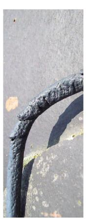
Figure 26: Examples of damages in cables in power plants located in the Atacama Desert.
