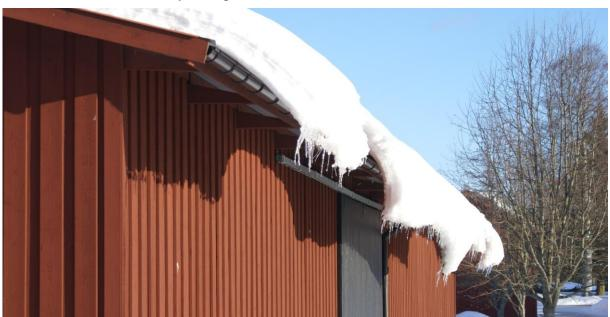
Figure 48: Picture taken on heavy snow and ice formation in spring in BJURÅS, Northern Sweden. Later, the frame showed a damage as in Figure 49 [Courtesy of Klaus Lorenz Högskolan Dalarna].
