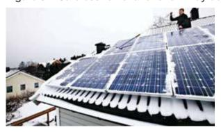
Figure 53: Brushing to remove snow from solar roofs [167].
