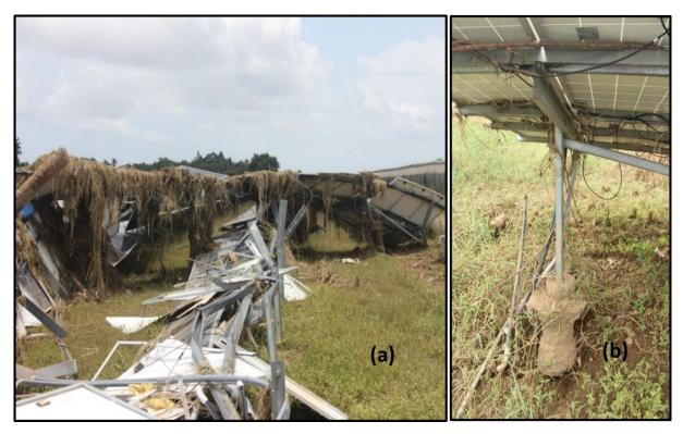
Figure 34: (a) Structural damage to PV plant P3 showing broken structures and modules. (b) An example where modules remained intact, but the foundations of structures were seen to be uprooted.
