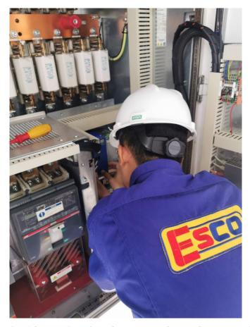
Figure 32: Regular checking and performing preventive maintenance in PV power plants in Thailand.
