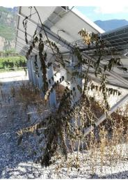
Figure 11: Growing bush in front of a tracker (left) and underneath an array (right) [Eurac Research].
