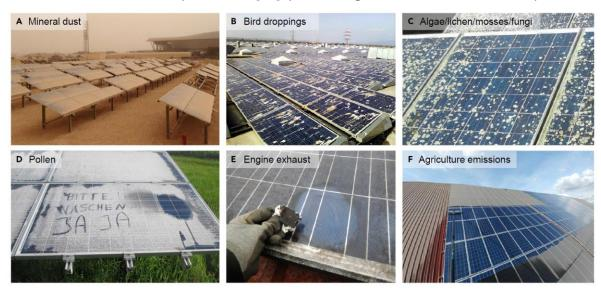
Figure 13: Examples of different types of soiling of PV arrays [83].
