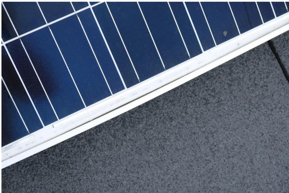
Figure 49: After winter, loose frames were observed on PV modules in Piteå in Northern Sweden [Picture from Mats Axelsson].
