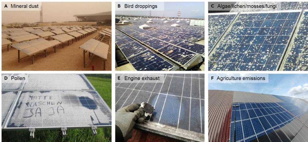
Figure 13: Examples of different types of soiling of PV arrays [83].
