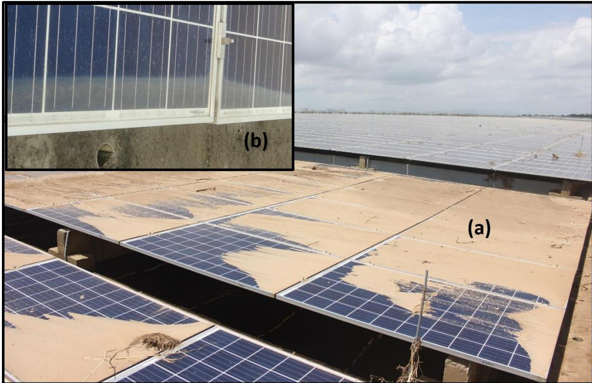
**Figure 36: (a) Silt was seen to be deposited post-flooding on most of the low inclination angle mounted modules in P2. (b) Uneven stains were observed near the bottom edge of most of the modules which could not be removed even after cleaning with soap water and scrubbing.**
