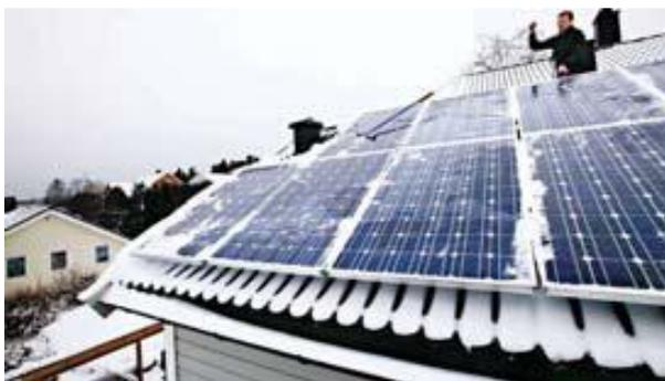
Figure 53: Brushing to remove snow from solar roofs [167].
