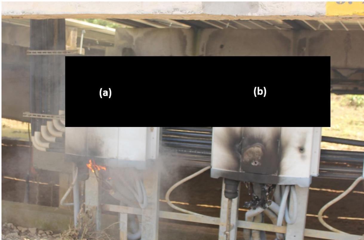
**Figure 40: (a) Fire was seen at an inverter several hours after the floodwaters had receded (b) A similar fire probably caused burn marks and failure of several submerged inverters. The manufacturer's name is masked in black.**
