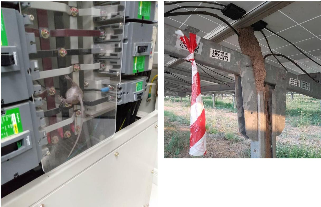
**Figure 30: Impact by wildlife on PV components, such as a rat in the main distribution box (left) and termites around the DC cable under the PV module (right).**
