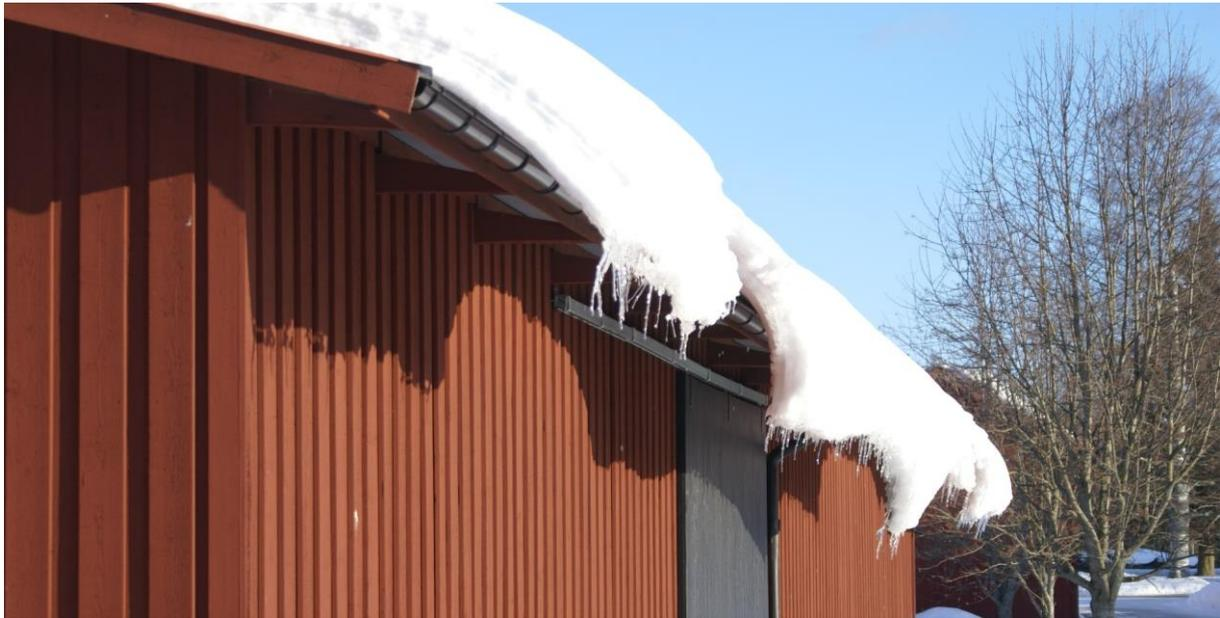
Figure 48: Picture taken on heavy snow and ice formation in spring in BJURÅS, Northern Sweden. Later, the frame showed a damage as in Figure 49 [Courtesy of Klaus Lorenz Högskolan Dalarna].
