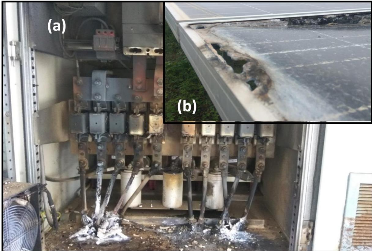
**Figure 41: (a) Damaged SCB due to submergence. Prominent burn marks are seen. (b) Even though the modules were not submerged, severe burn marks that cause the melting of module glass were seen near module edges.**
