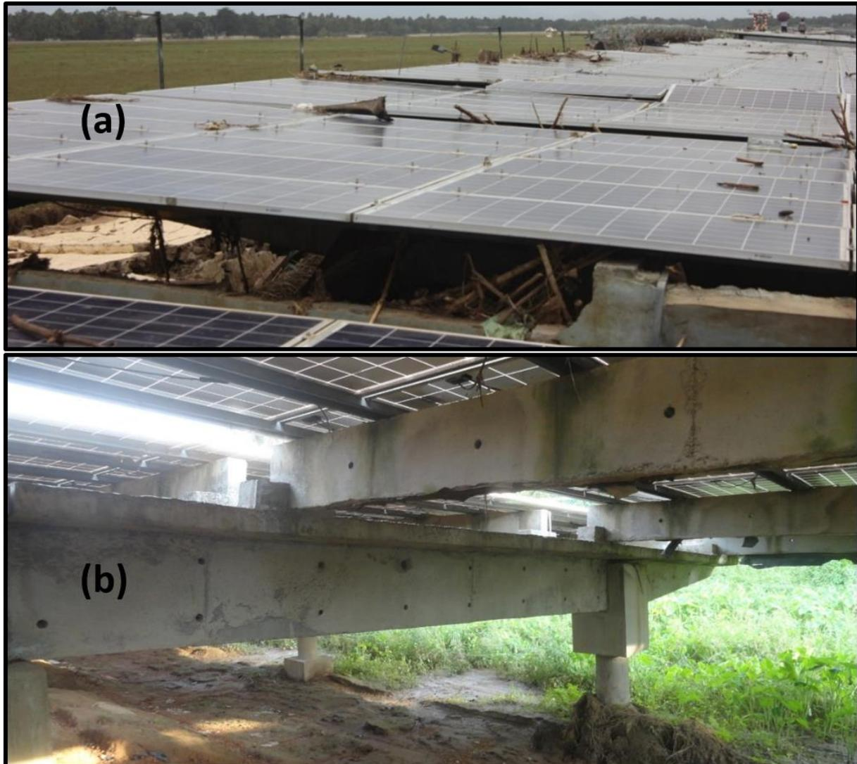
**Figure 35: (a) Top view of Canal top plant P2 showing that hardly any damage to modules or structures was seen despite this plant being submerged under fast-flowing water. (b) Bottom view of the all-concrete structure of P2 showing concrete beams.**
