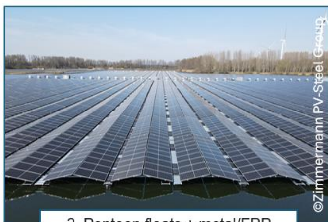
2. Pontoon floats + metal/FRP (examples: Scotra, Zimmermann)
