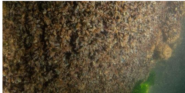
f) Biofouling of underwater component [76]
